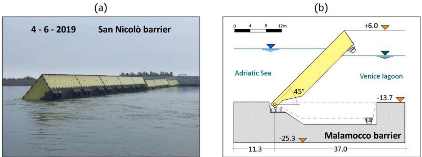
Fig. 2. Mo.S.E. system. (a) view of the flap gates of the San Nicolò barrier partially raised under the test of 4 June 2020 (photo by R.A. Mel); (b) working position of a single flap gate of the Malamocco barrier (data in meters and elevations referred to the PS reference datum).
